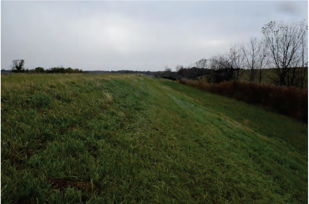
West downstream slope
