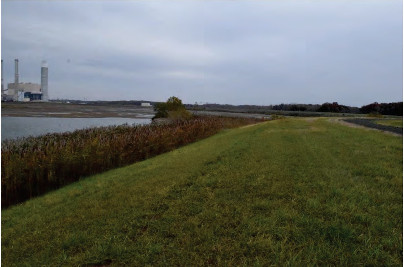
East crest and upstream slope
