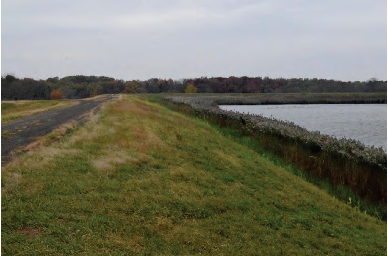
South upstream slope and crest
