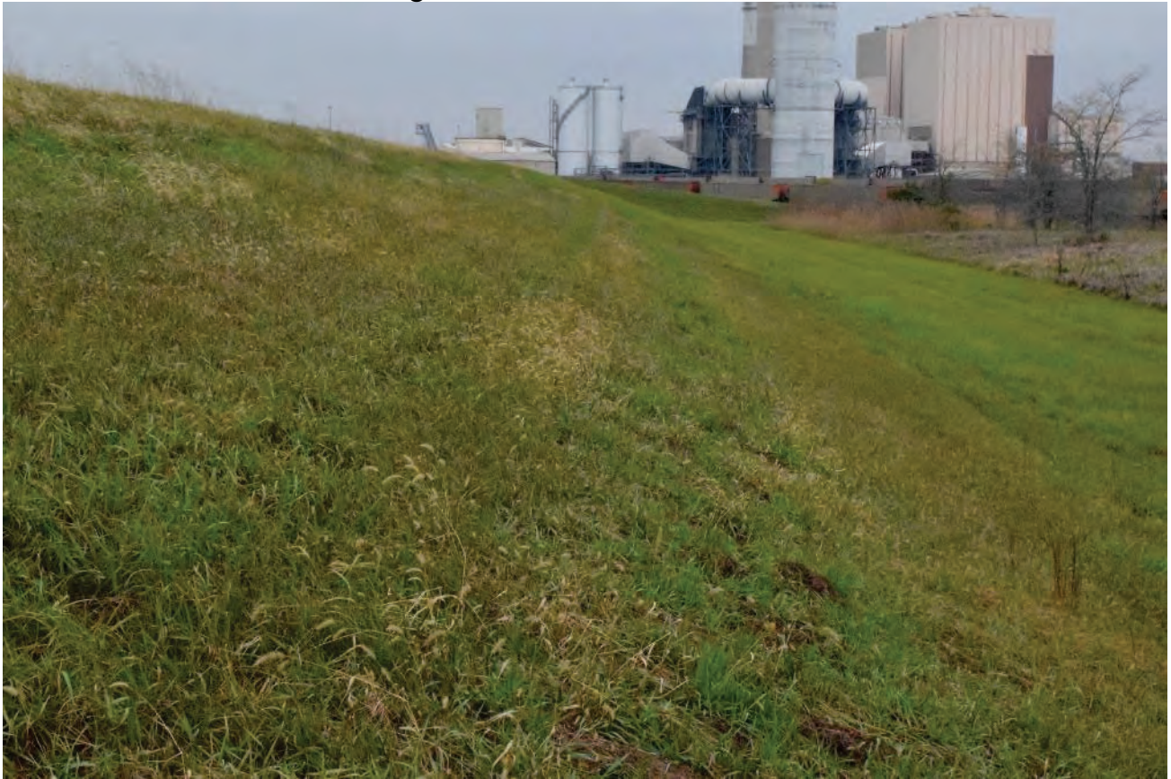
North downstream slope
