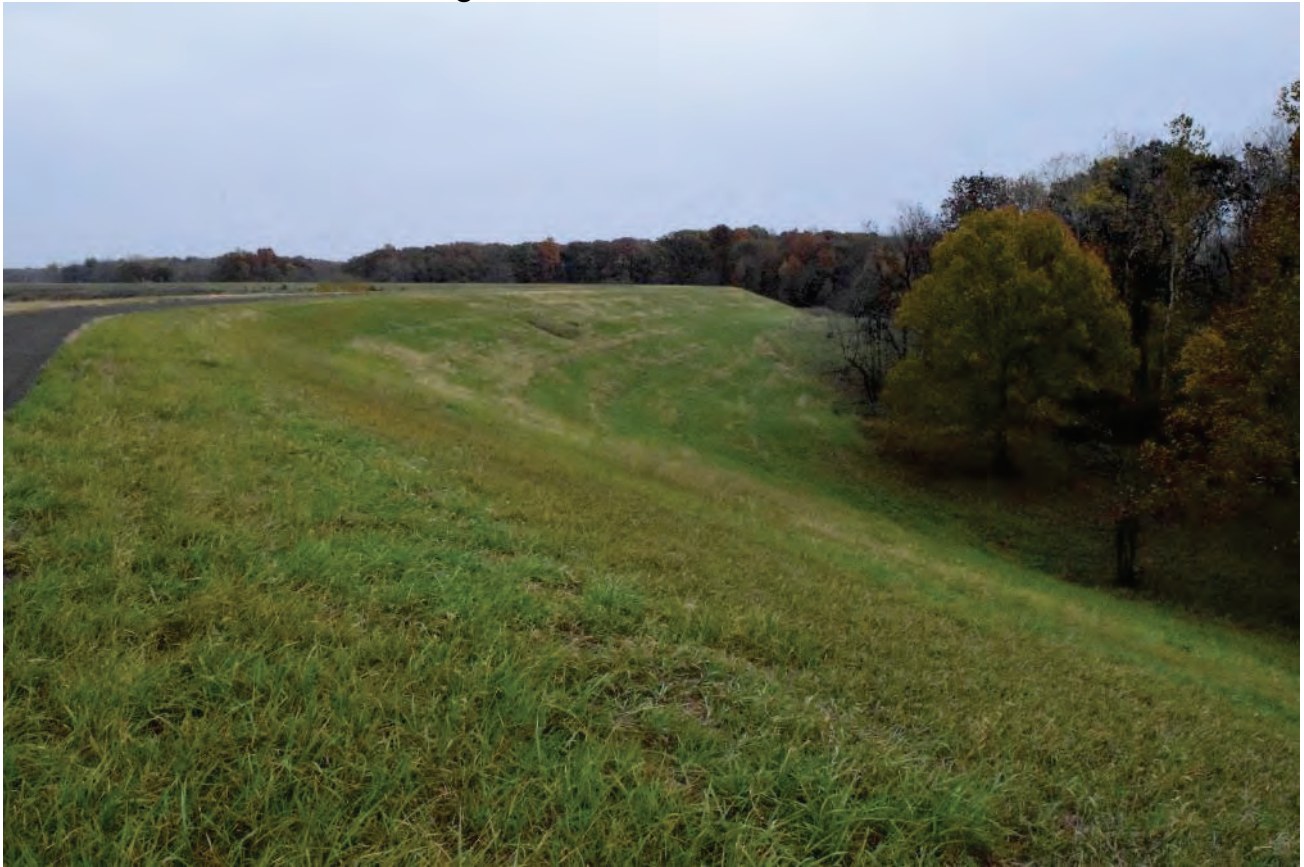
East downstream slope
